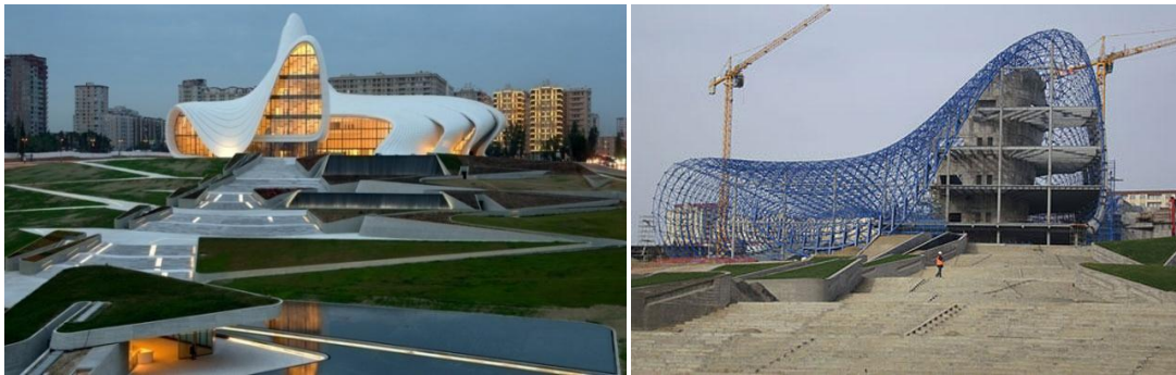
Figures 8. 9. Haydar Aliyev Cultural Center, Front and Construction Views (17-18)
