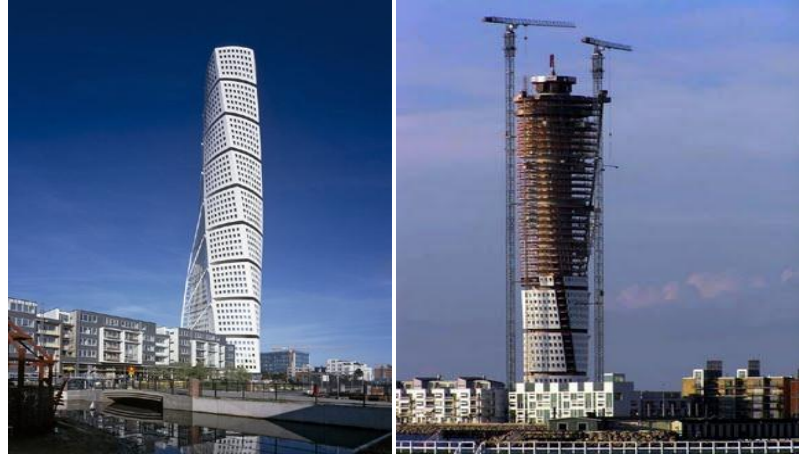
Figures 16. 17. Turning Torso Tower View and Construction View (27-29)
