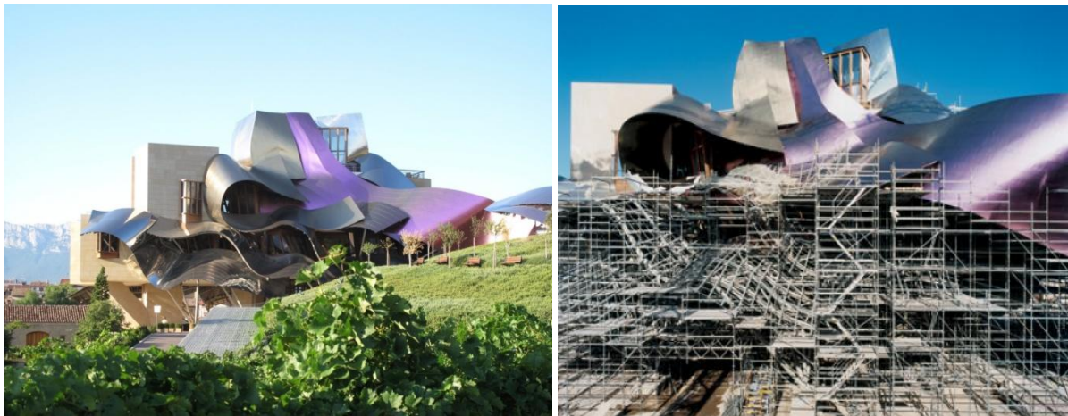
Figures 5. 6. Marque de Rascal Hotel, Front and Construction Views (12-13)
