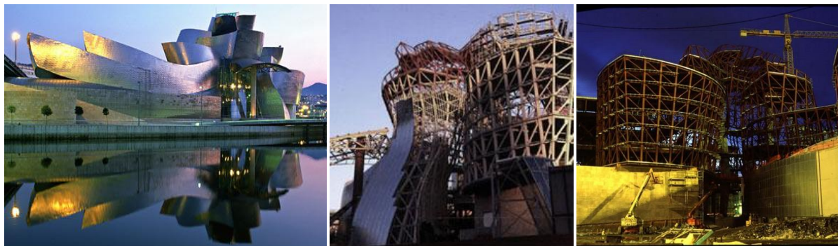
Figures 1. 2. 3. Guggenheim Museum Bilbao Front and Construction Views (8-9)
